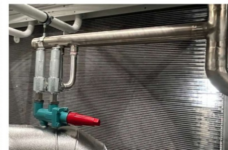
Safety valves on LP side (set 16 bar)
